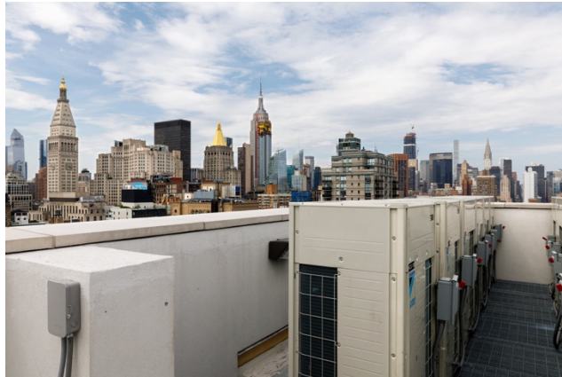
Some of the mechanical equipment for the building's variant refrigerant flow heating-and-cooling system, which can be twice as energy efficient as more conventional systems. Stefano Ukmar for The New York Times
