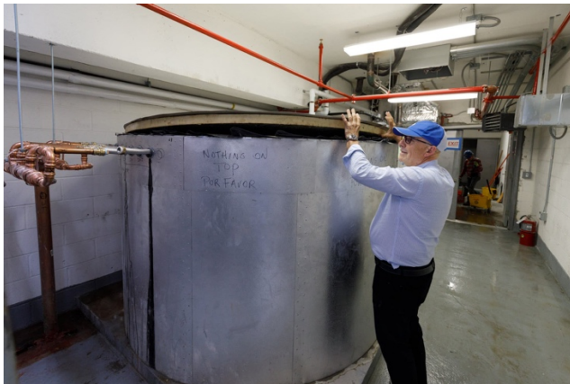
The developer, Michael Namer, in a mechanical room with equipment that helps heat the building's potable water with solar energy. Stefano Ukmar for The New York Times
